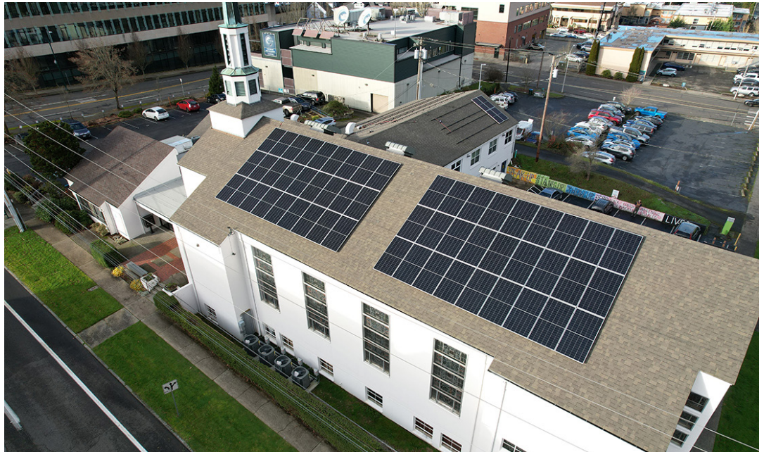
Drone view shows new solar panels installed at United Churches of Olympia.
