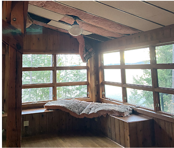
Rory McDonald repaired metal roof on Forrester Lodge and inside insulation and tiles from leaks. Photo by Leah Atkinson Bilinski
