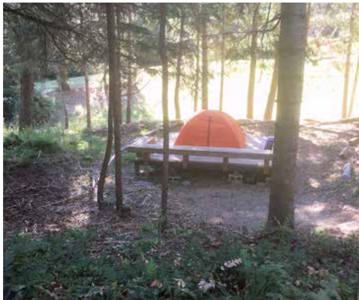
Tenter uses one of two new tent platforms at N-Sid-Sen, built with wood from Cabin 8, which was damaged by a fallen tree.
